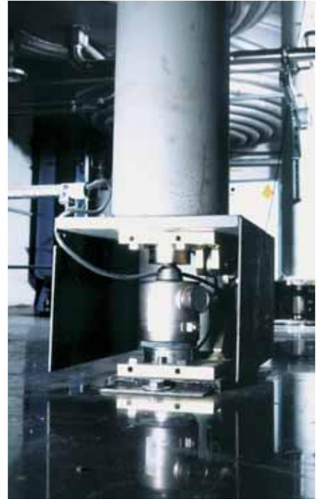
Tank and hopper weighing
